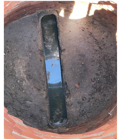
Photo of a Manhole
