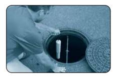
iTracker smart sensor installation is accomplished in 20 minutes without the requirement for confined space entry. Simply hang the sensor weighing less than 2 lbs. from a factory supplied spanner bar, via Bluetooth enter manhole number, pipe size and water level into the calibration screen displayed on your mobile phone and the iTracker is ready to begin collecting data. It's as simple as that!
